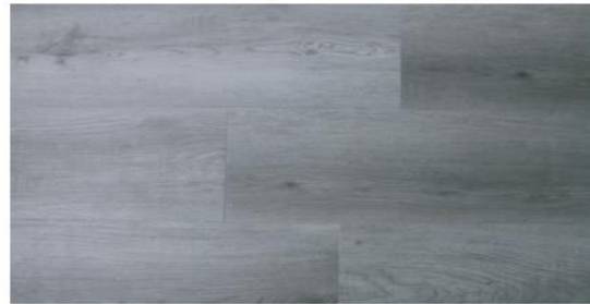
5 When the installation finishes, the floor is flat and does not have aperture. if the floor are not smooth or have slit, they need to be lifted slight and locked them by 10-30°angle. After locking, floor would be smooth automatically.
